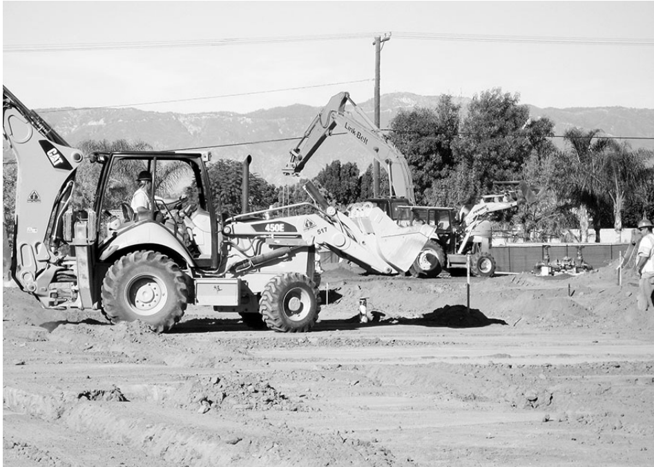
Tractors and machines are shown installing the underground lines.
