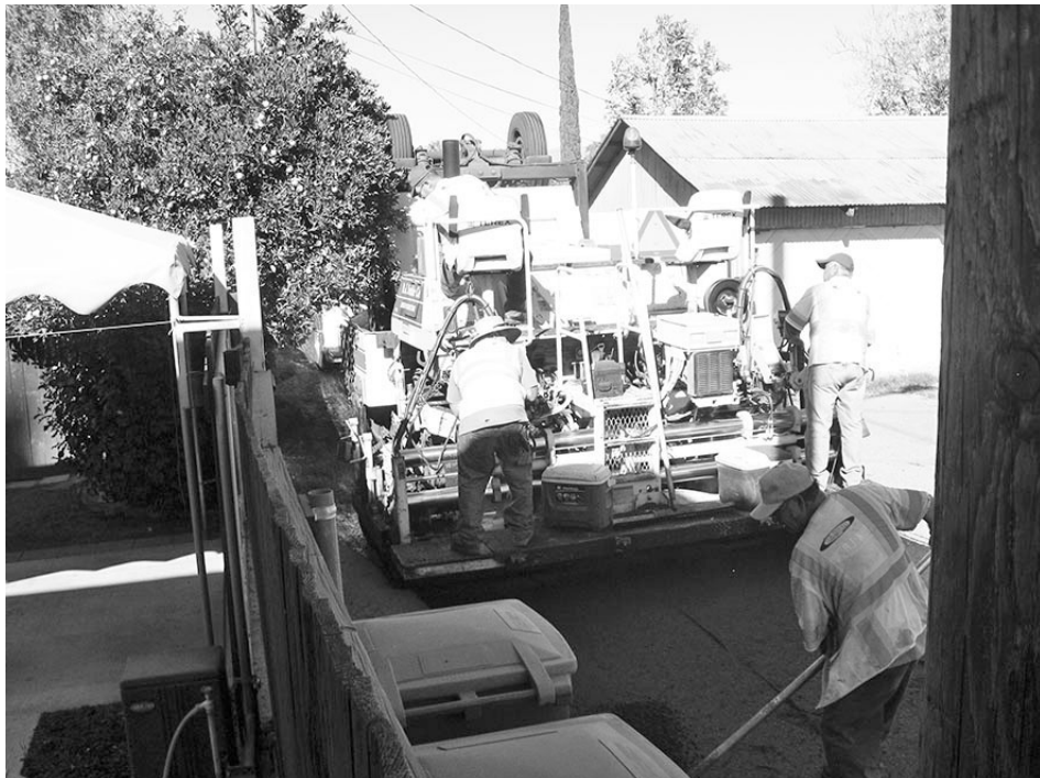
Workers fine tune the edges by hand behind the paving machine.
