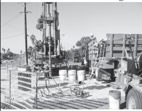
The Northwest corner of Center and Iowa Ave. has been undergoing drilling where samples of dirt are being removed and put into barrels for testing. The City of Riverside has contracted with the drilling company from Montclair When these pictures were taken on Nov. 16, 2010, the core samples were being taken from a depth of 120 feet.
