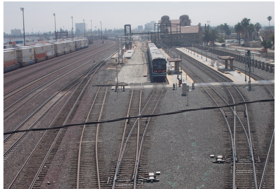
The railroad yard is on the left and Metrolink tracks are on the right.
