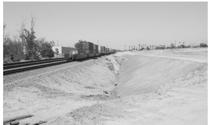
New dirt roadway across the arroyo (no drain pipe)
