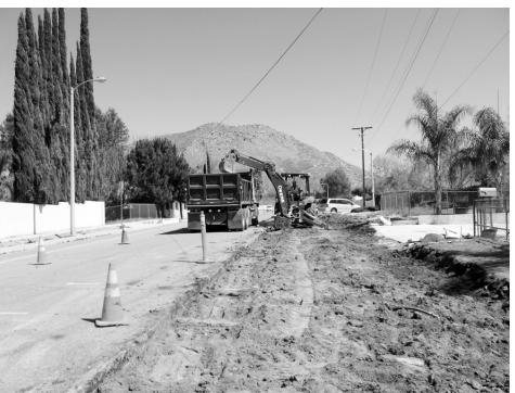
The old asphalt was removed and hauled away by dump trucks to widen Main St. on the Riverside County side of the county line. 300 feet of new asphalt, curb and gutter, a sidewalk and 4 driveways were added between Michigan and the Highgrove Community Park entrance at an additional cost of \$41,795.00 according to Juan Perez of the Riverside County TLMA.
