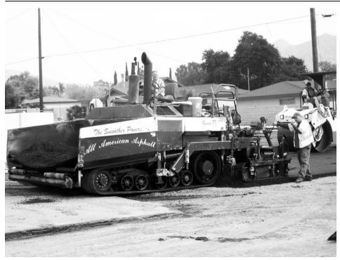
The base coat of asphalt paving was done on Saturday March 24, 2012 and there were a lot of large trucks carrying asphalt to this paving machine. New base was laid on Main St. between the Highgrove Community Park and Sanrive and on Michigan on both sides of the count line.
