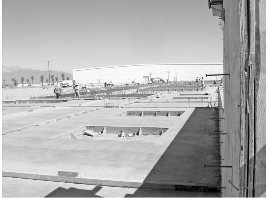
This view shows the new wall that will be tilted up and become the east wall of the new Sabert Corp. addition. The existing building in the distance is the rear of their building that is located at 860 Palmyrita Ave. between the Union Pacific railroad track and Northgate and just east of the new Dole warehouse.
