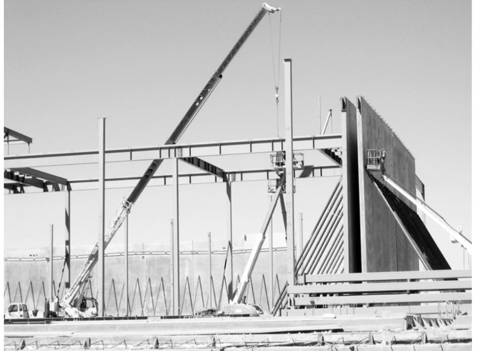
This large crane lift the steel beams into place assisted by smaller cranes.
