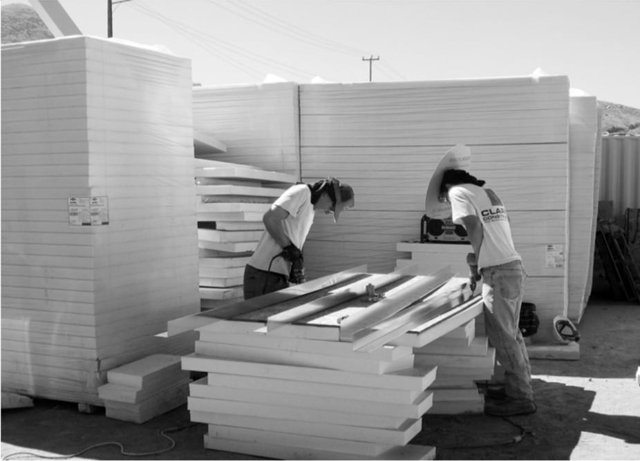
These workers are putting framework around the insulation. It was very hot that day so the man on the right made a hat for shade out of a piece of cardboard.
