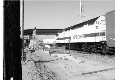
Overhead beams for Iowa Ave. overpass placed over the tracks!
