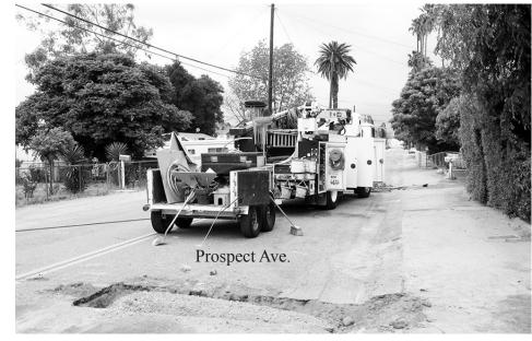
Various old water lines are being replaced in Highgrove and water meters are being relocated by City of Riverside Public Utilities.
