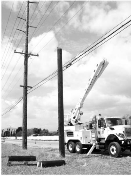
On Feb.27,2012, the crew shown above was in the process of adding crossbars to the tall electrical poles to hold the electrical wires along Spring Street. The shorter poles are being removed. The tall heavy duty poles were installed to get power to the Spring Mountain Ranch area a few years ago when the economy was much better.
