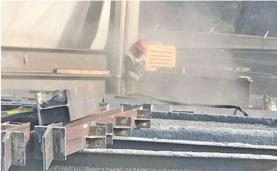
The photo above shows the metal beams being blasted and the dust it creates on the north side of Main Street.
