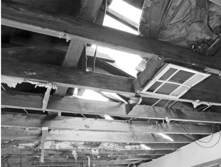
This is an inside view of the same hole that was cut in the roof by firemen to gain access to the fire. This photo was taken on Dec. 28th., 2 days later.
