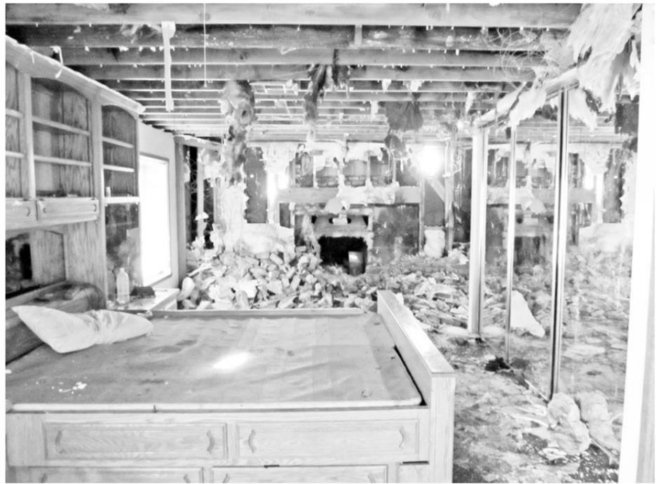
The upstairs bedroom had extensive damage to the ceiling, roof, and trusses and there probably was water damage to both the top and bottom levels. This is the view of the upstairs bedroom. The bricks from the wall had to be removed to allow firemen access to the wall that was smouldering.
