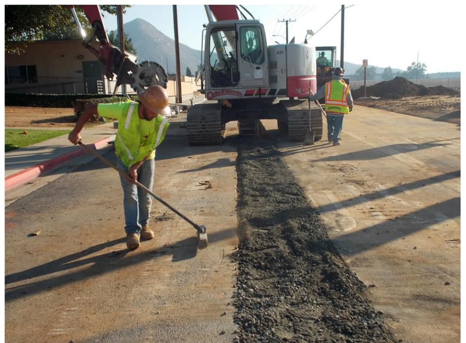
This view shows workmen by the school on Garfield covering up the new sewer line that will tap into the existing sewer line along Center Street.
