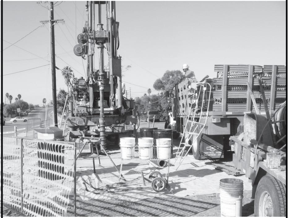
The Northwest corner of Center and Iowa Ave. has been undergoing drilling where samples of dirt are being removed and put into barrels for testing. The City of Riverside has contracted with the drilling company from Montclair When these pictures were taken on Nov. 16, 2010, the core samples were being taken from a depth of 120 feet.
