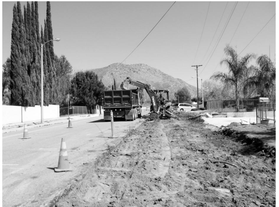
The old asphalt was removed and hauled away by dump trucks to widen Main St. on the Riverside County side of the county line. 300 feet of new asphalt, curb and gutter, a sidewalk and 4 driveways were added between Michigan and the Highgrove Community Park entrance at an additional cost of \$41,795.00 according to Juan Perez of the Riverside County TLMA.
